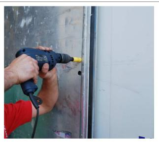
Milling and eliminate any ridges or edges inside the counterbore in order to properly position and align the spacer. Below, the picture shows the final configuration (side of the cone from the inside).
